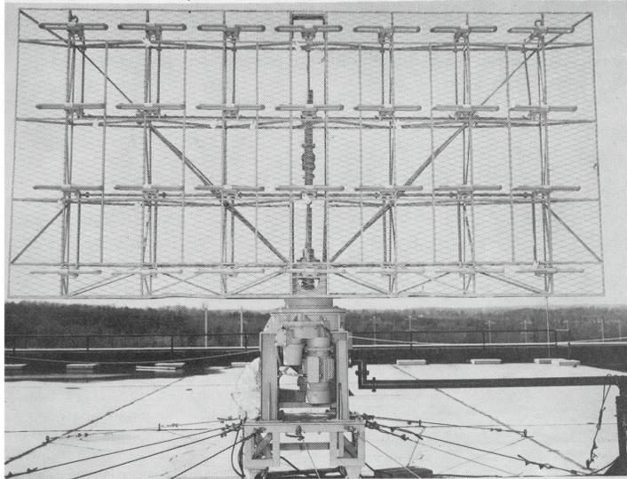
**Figure 3-15.—Bedspring array.**
