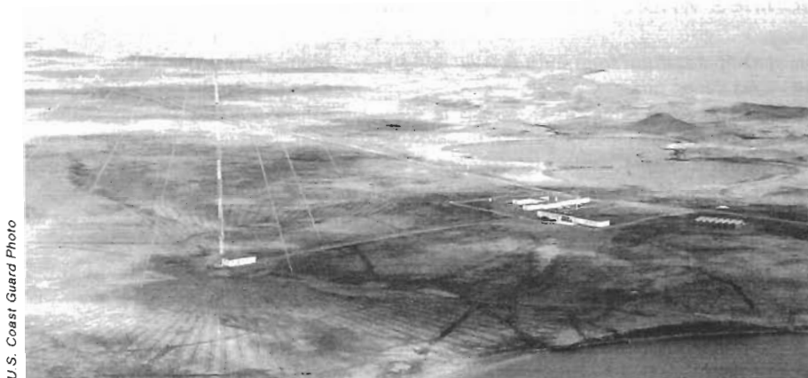
LORAN-C transmitter at St. Paul Is., Alaska, has a 625-foot antenna.
