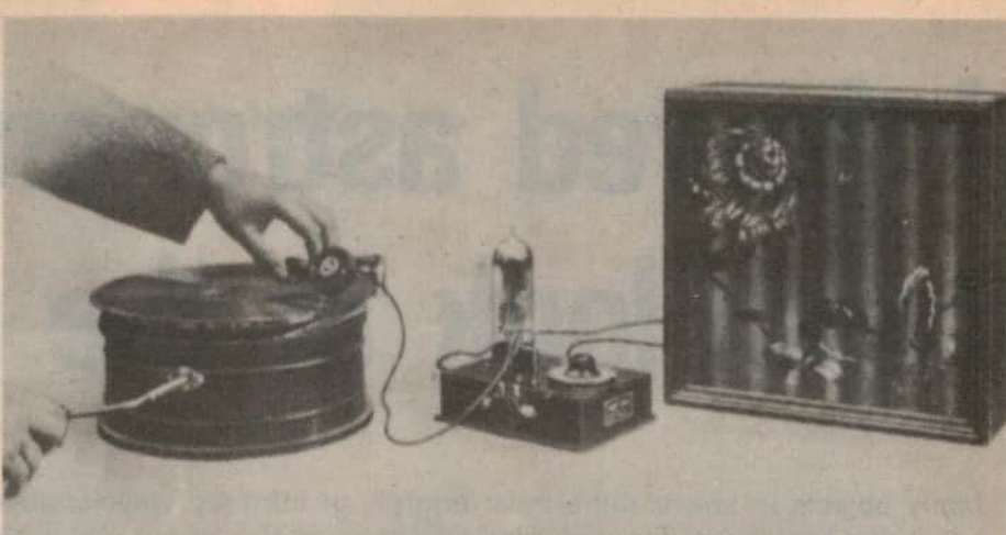
Fig. 4: a 1928 version of the OE333 in use as an amplifier for record playing equipment. Note the hand-cranked turntable.
