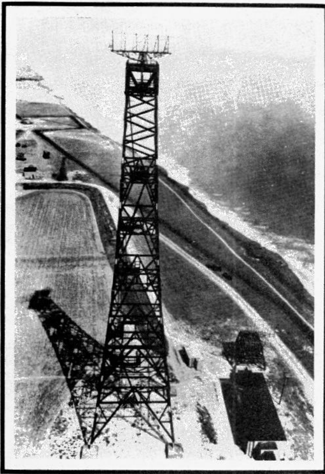
Fig 3. A coastal defence tower. Standing some 360 ft high, the apparatus was used to detect low flying intruding aircraft which were flying too low for normal stations to detect them. Lone raiders often adopted this tactic to reach specified targets, or to make photographic records.
