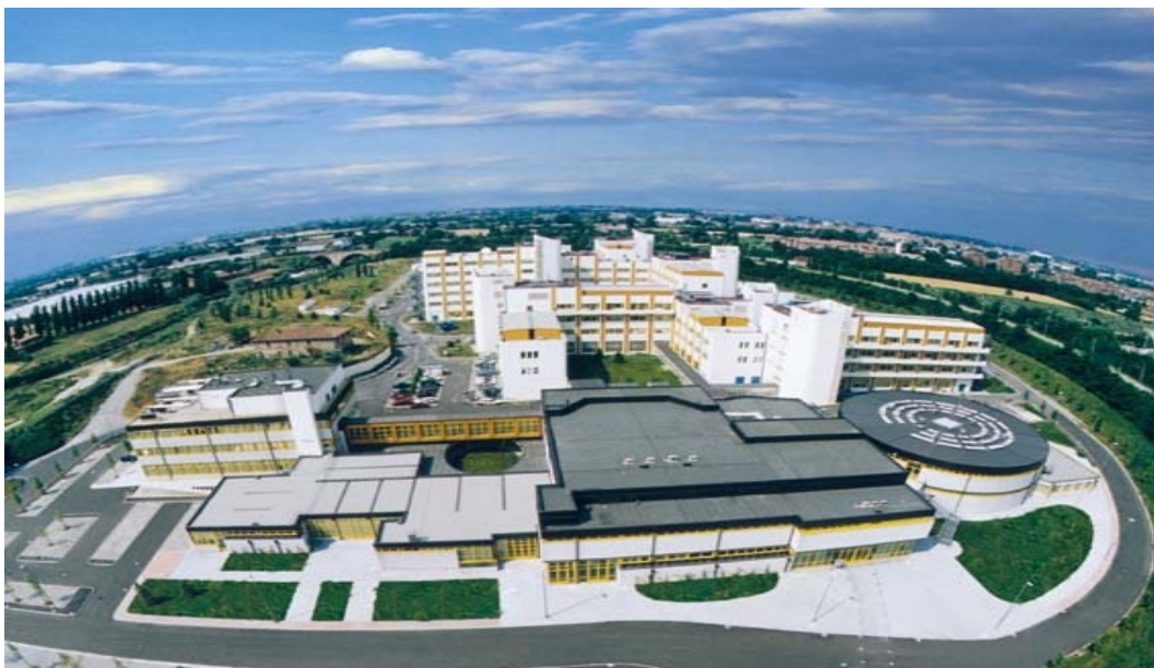
Figure 2.8. CNR campus in Bologna, Italy (courtesy of CNR).
