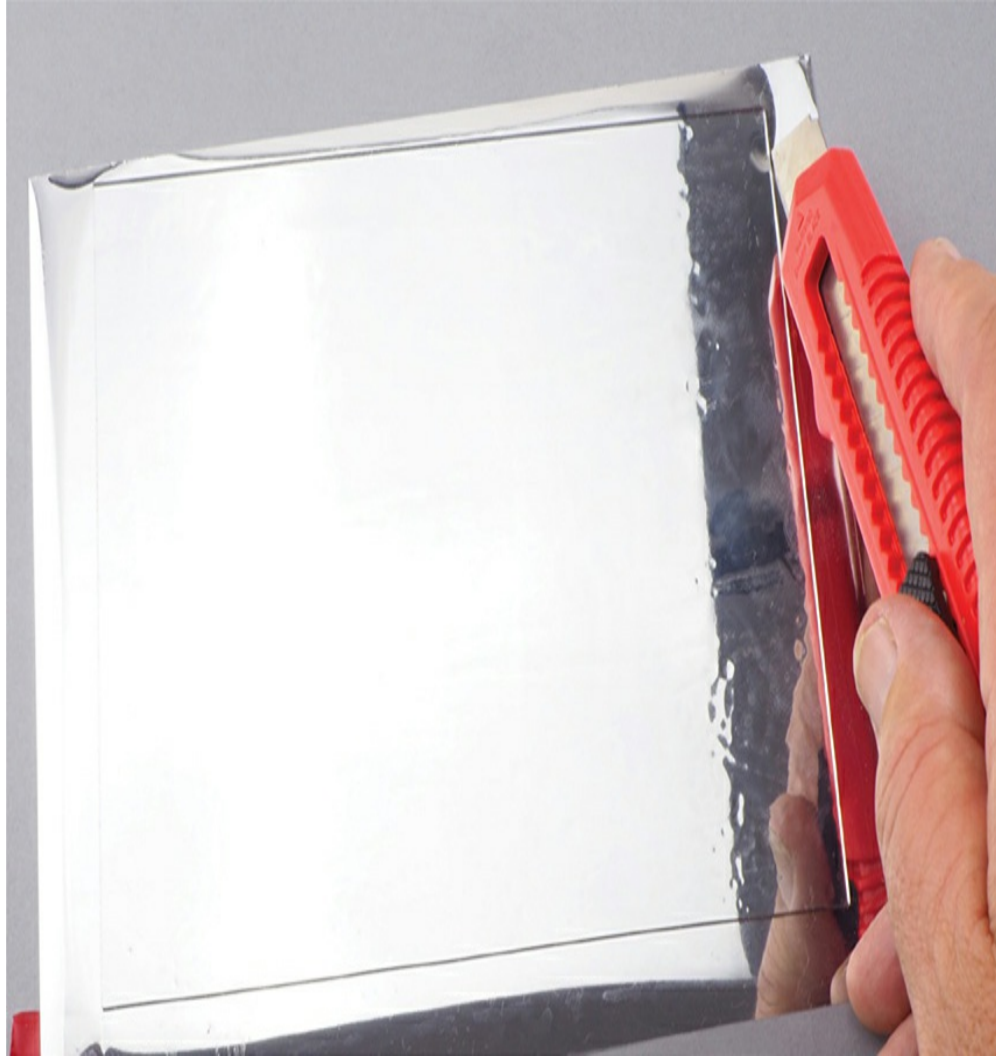
Figure 3-16: Trimming the reflective window film
