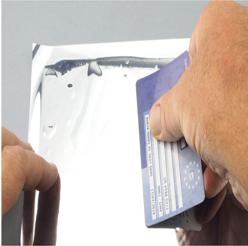
Figure 3-15: Removing bubbles from the reflective window film
