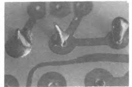
The two joints shown here are typical of a case where the solder tip and components being soldered are not brought together at the same time. It is also apparent that not enough solder has been applied.
