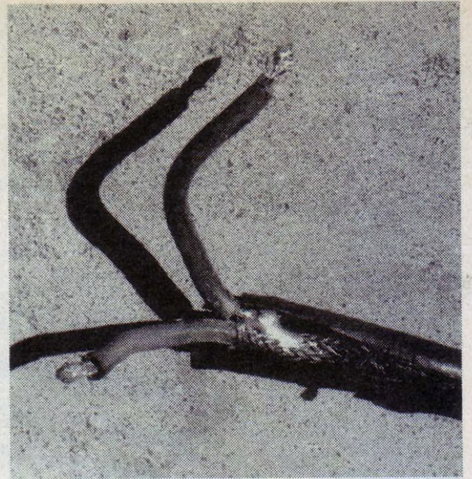
This photo shows the troublesome shielded wire in the old HMV radio. The short circuit was at the solder joint where the heat of the soldering iron had damaged the rubber insulation of the inner lead. This problem has been encountered before in other old receivers, so it was not an isolated incident.
