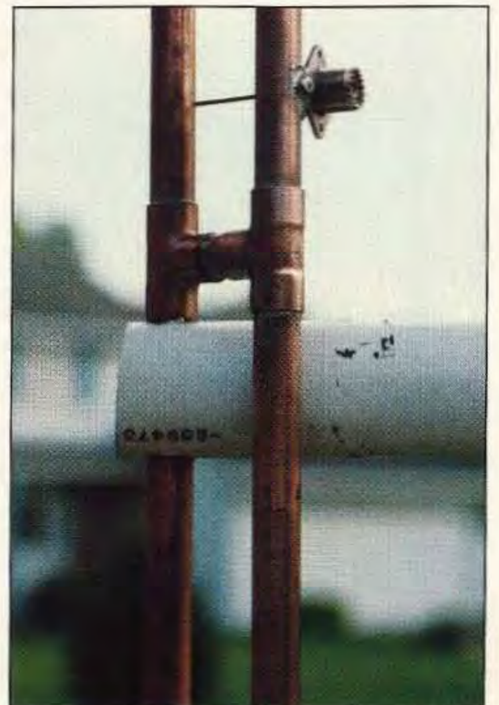
Photo B. Run the long section of the Double Cactus through the PVC pipe to secure it to the tower side mount.
