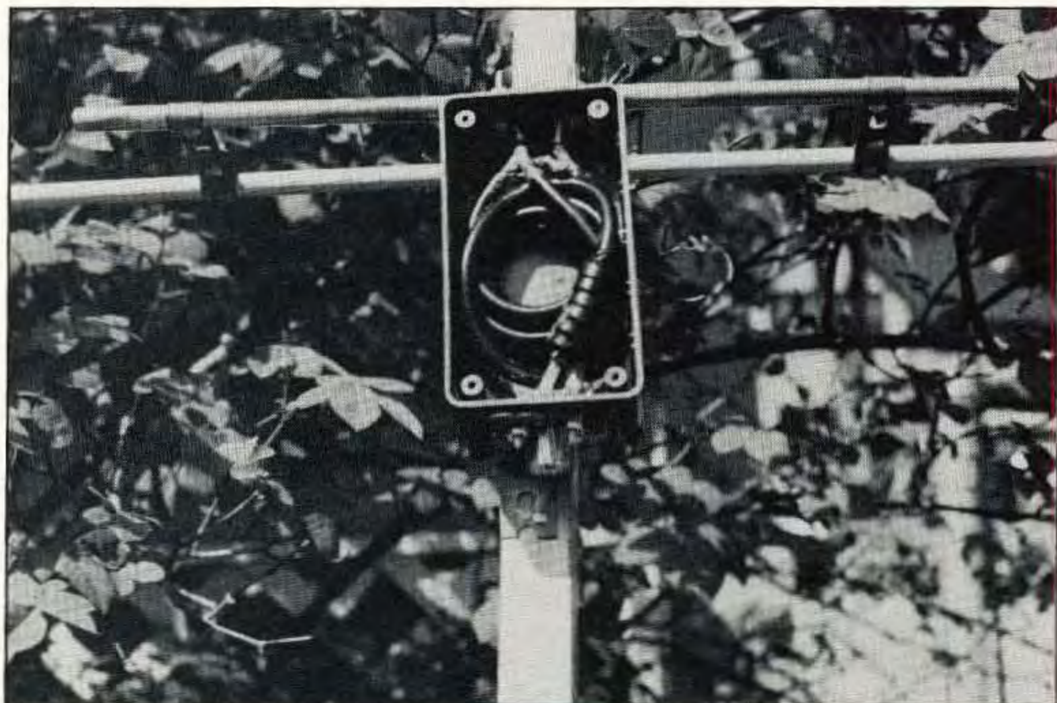
Photo B. Close-up of balun box. Note the "T" match bars and the driven element.
