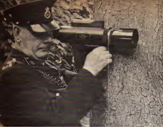
A police observer using a hand-portable passive sight infra-red viewer
