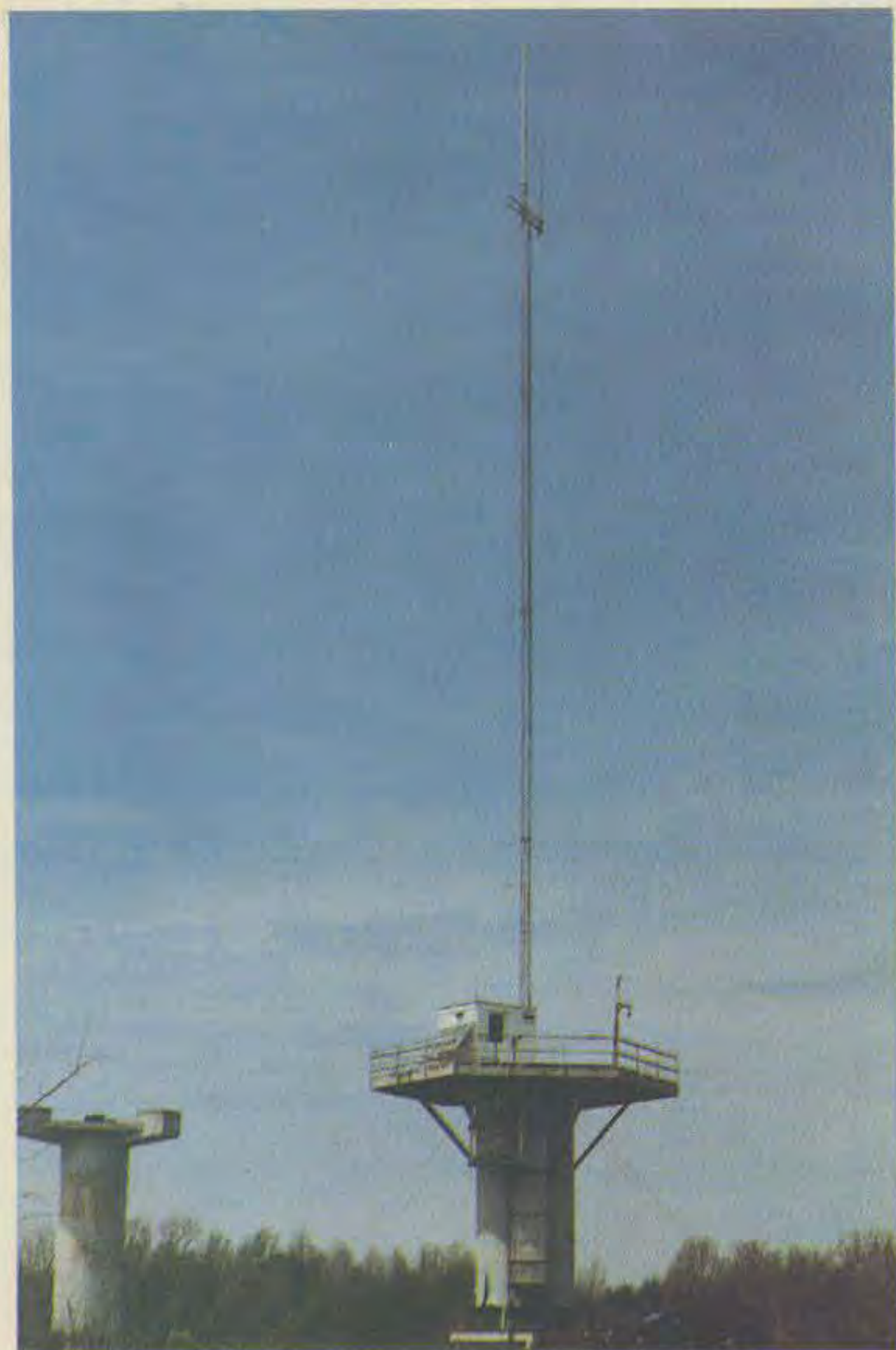
Photo A. AARC repeater. Photovoltaic array is visible on the left side of the shack at the base of the tower.
