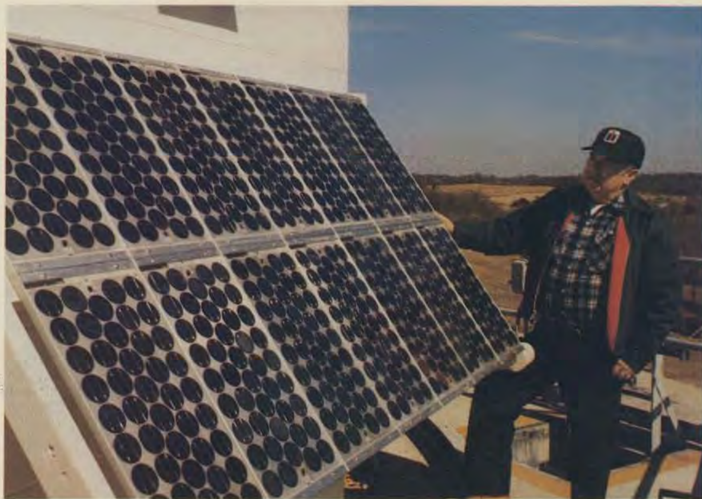
Photo B. Photovoltaic array. Frank Troutman WB3CLF helped install the array on the side of the shack.
