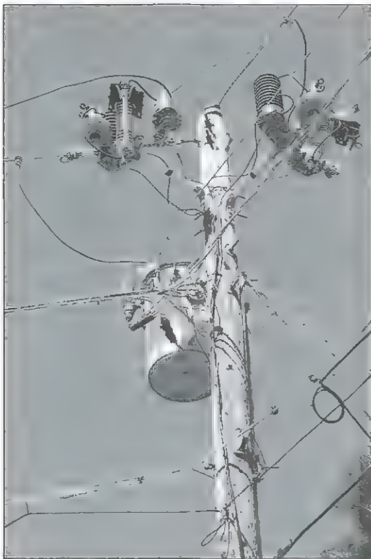
Figure 9.11 — Utility poles and power lines must be given wide clearance from your antenna system.
