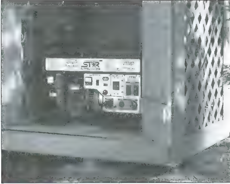
Figure 9.6 — Install your generator in a well ventilated area, away from living areas.
