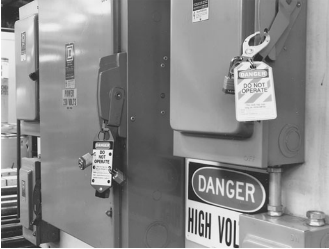
FIGURE 2.57 Typical application of locks, tags, and multiple-lock devices. (Courtesy Ideal Industries, Inc.)
