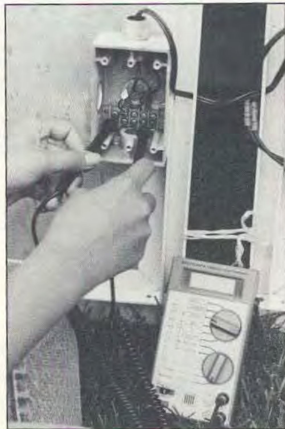
Photo B. Test the panel, using care to observe the polarity of the panel output.
