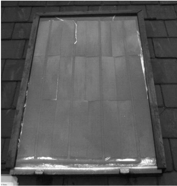
Figure 4-7 A home-made clip fin collector.
