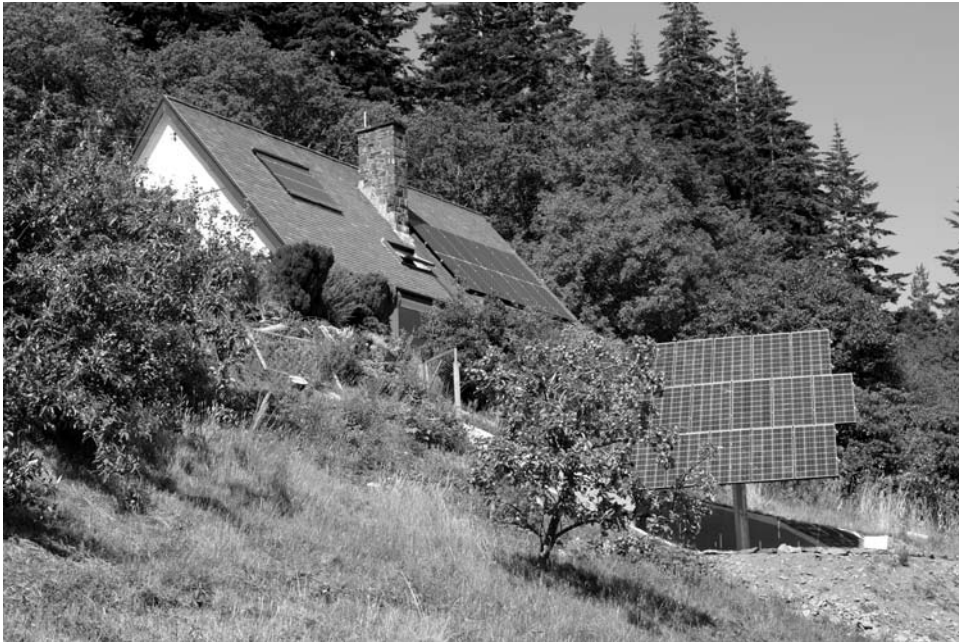
Figure 14-2 Solar tracker at Llanrwst, near Snowdonia, Wales. Image courtesy Dulas Ltd.
