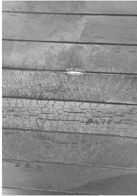
Figure 8-3 The burnt hull. Image courtesy Massachusetts Institute of Technology.
