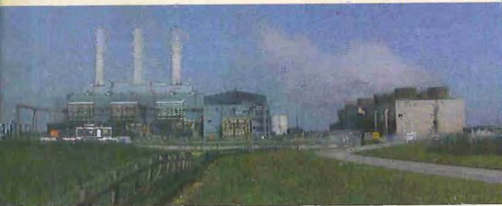
General view of the Killingholme "A" Gas-fired Power Station.
