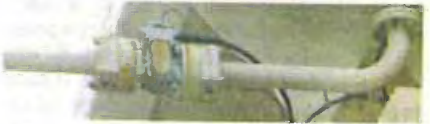
A Buchholz, safety switch, relay is fitted on oil-cooled transformers and detects any build-up of gases in the oil.
