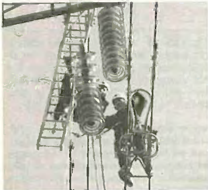
National Grid engineers installing glass insulators on an overhead cable.
