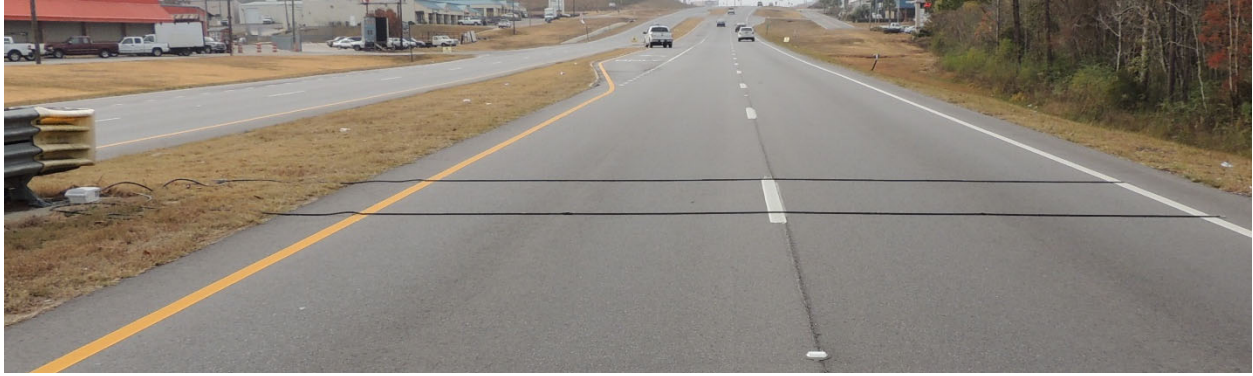
FIGURE 1 Example of road tubes installation. (Image Credit: Marcus Brewer)
