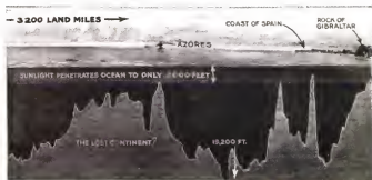
Fig.7: the ocean floor between Newport, Rhode Island (USA) and Gibraltar, as determined by the USS Stewart in 1922. This survey used the Hayes Sonic Depth Finder and found what was thought at the time to be the lost continent of Atlantis. From Popular Science, May 1923.
