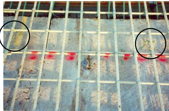
Figure 4. Chair Placement for GFRP Reinforcement.
