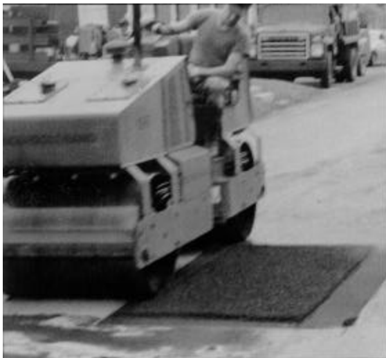
Figure 3.11. Overlapping compaction lanes
