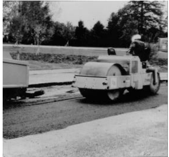
Figure 3.10. Steel-wheel roller
