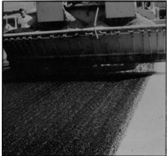
Figure 5.2. Applying aggregate with self-propelled hopper-type spreader
