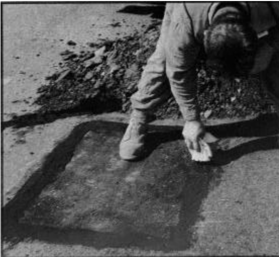
Figure 3.13. Sealing edges of the patch
