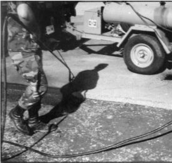
Figure 3.7. Applying tack coat with spray wand
