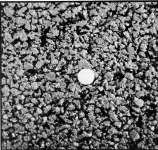
Figure 8.1. View of a porous friction surface (PFS)
