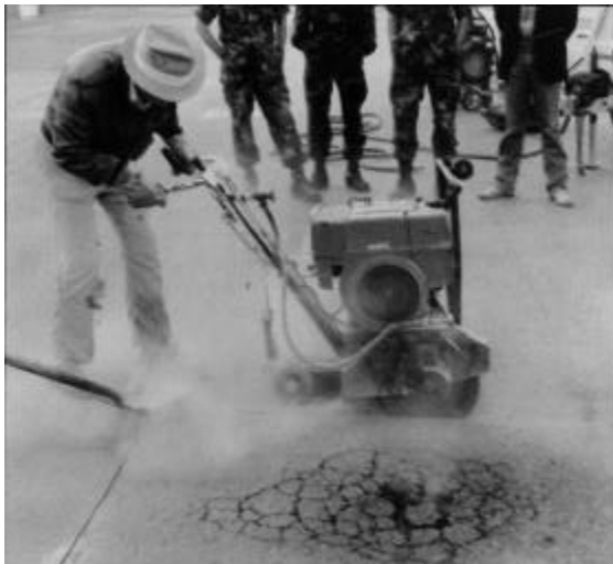
Figure 3.3. Saw cutting marked repair area
