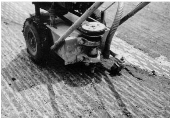
Figure 6.1. Vertical spindle router
