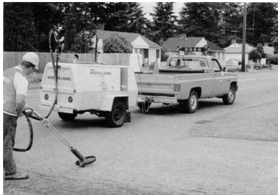
Figure 6.6. Hot compressed-air heat lance
