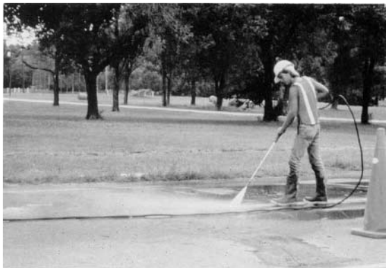
Figure 6.5. High-pressure water cleaning equipment
