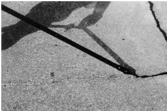
Figure 9.3. Sealing the crack
