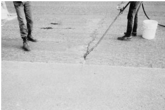
Figure 9.1. Filling crack with sand emulsion mixture
