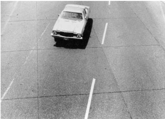
Figure 3.1. Example of reflective cracking
