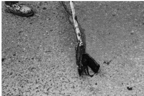
Figure 9.4. Using a squeegee to remove excess sealant
