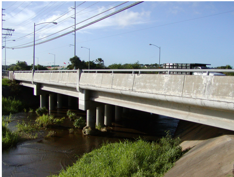
Figure 5-8: Elevation of typical AASHTO-type girder bridge
