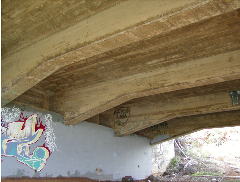
Figure 5-5: T-beam girders with sloped soffits
