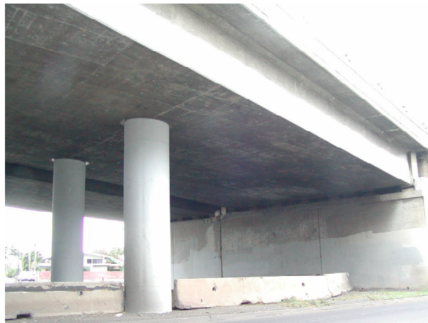
Figure 5-12: Typical multi-cell box girder bridge
