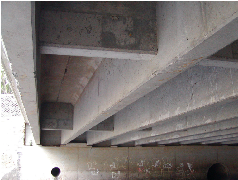
Figure 5-3: Elevation of typical T-beam bridge
