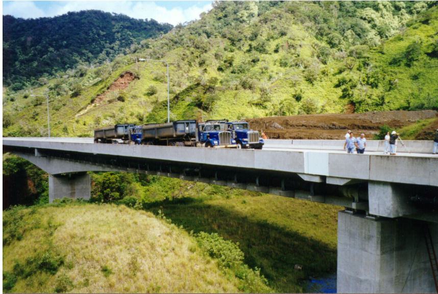
Figure 7-1: Load-test on the North Halawa Valley Viaduct
