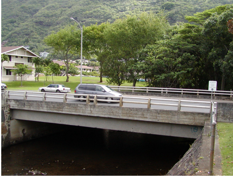
Figure 5-3: Elevation of typical T-beam bridge
