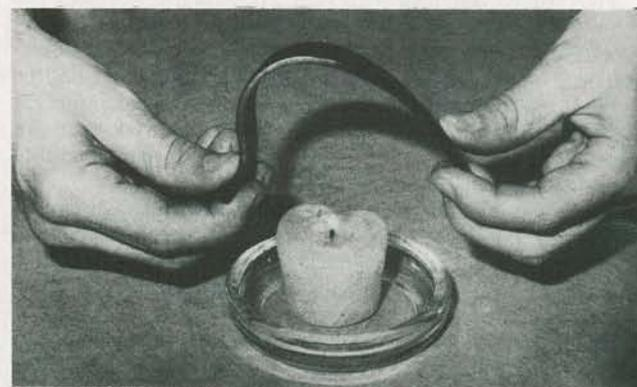
FIG. 3—ACRYLIC PLASTIC CAN BE EASILY BENT into any shape, if it is heated.
