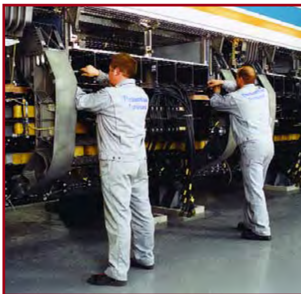
Figure 5. Under the covers of the propulsion and guidance system of the Transrapid train. (Source: Siemens AG)
