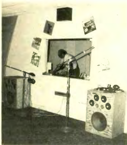
Asbury Records' studio features heavily carpeted flooring and semi curved walls (left) to inhibit sound reverberation. The glass pane in the studio-to-control room window is tilted slightly for additional protection from reverb. Microphones are attached to booms to insure exact positioning during recording sessions. The dual multi-coned speakers on either side of the control room window are used for playback of recordings. A row of microphone connectors seen between the two boom mics lead directly to the control room mixing console on the other side of the wall. Album covers serve as decoration around the control room window.
