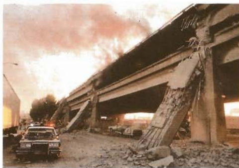
DON'T LET THIS HAPPEN TO YOUR EQUIPMENT: Prepare for earthquakes—they occur all over the world.
