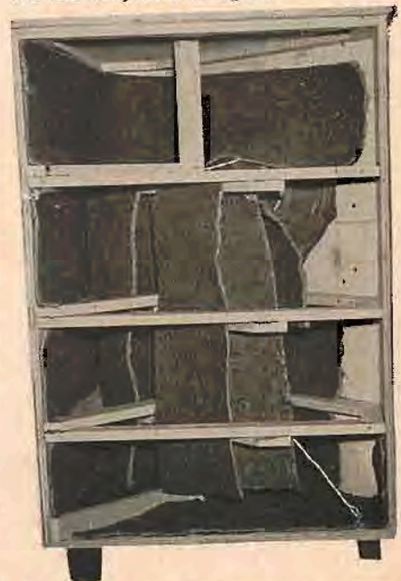
Fig. 4. Scrap strips of Ozite lining are draped over internal bracing to further dampen the cabinet.
