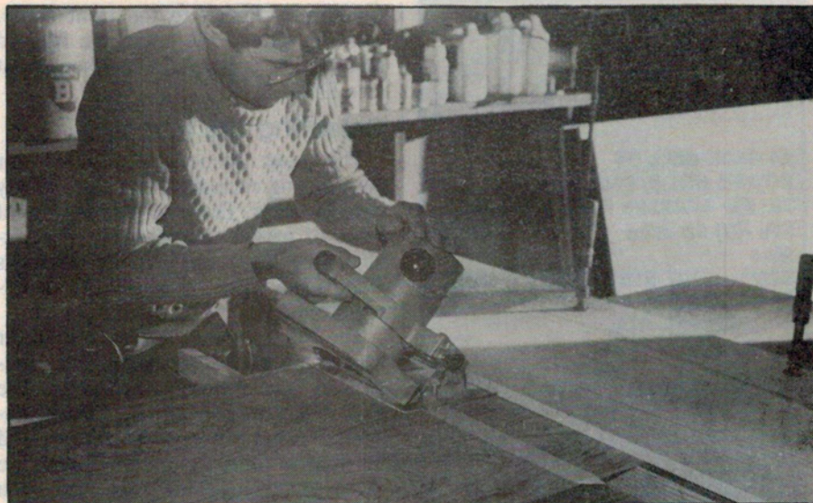
Photo 2: accurate mitre cuts can easily be made by clamping a straight plank to the panel and using this to guide the sole-plate of your power saw.
