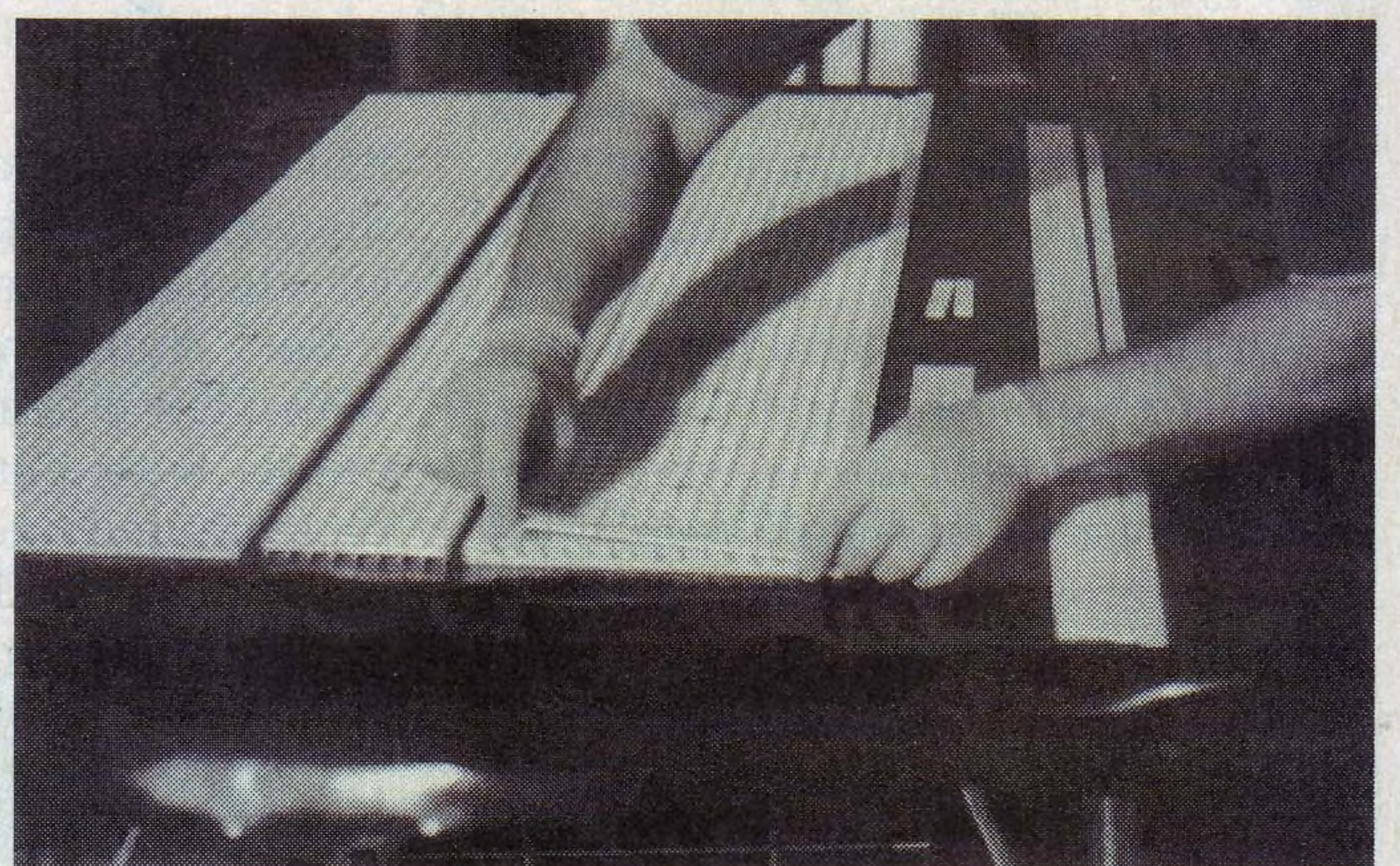
After glue has been applied to the top of the matrix panels, the air gap spacers are placed around the periphery, as shown here.
