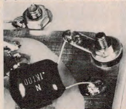
The 0 V track on each module pc board is 'earthed' via a 100n greencap to the earthing bolt, which is first insulated from the board using a transistor mounting insulator. (See also page 34).
