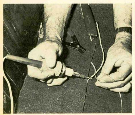
Solder and tape these leads to a main wire that will join all mat leads together. Then, route this main wire underneath the carpet to the spot where the central alarm model will be located.
