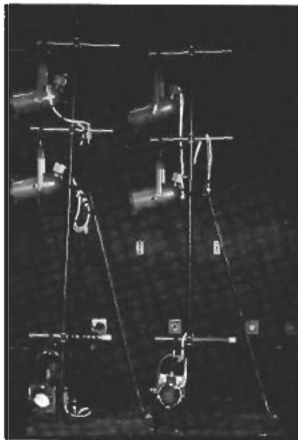
Figure 5. Reinforced light towers designed for asymmetrical loading.
